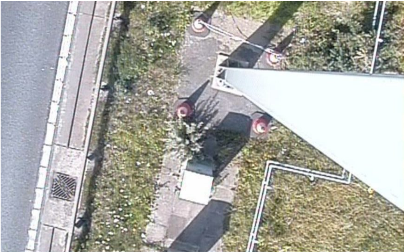
Eyes down: a camera on the M6 is found to be pointing at the ground
